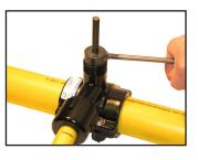
**16** To allow flow through service, back punch up until the top of the punch is flush with top of saddle. It is important that the punch does not protrude above the top of the saddle tee.
