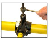
**11** Tighten the compression nut until it shoulders against the outlet. Do not overtighten. **CAUTION:** To prevent inadvertent pull-out of the P.E. tubing during the assembly process, complete step 11 immediately after step 10, without delay and ensure work is not being performed on the free end of the P.E. tubing.
