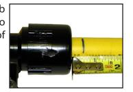
**15** Screw punch down until stop on drive key contacts the top of the saddle tee. The tap is now complete.
